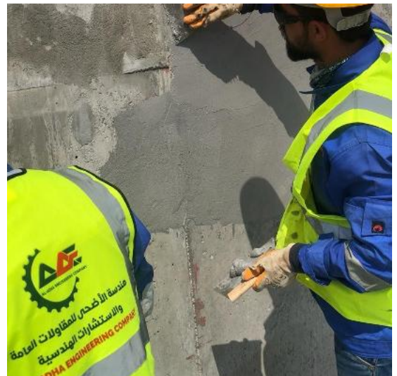
Concrete repair and surface-treatment works.
