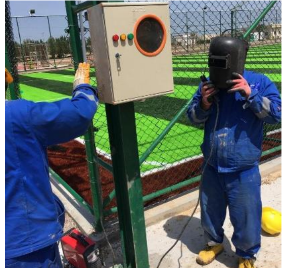
Sports-field fencing and lighting installation.
