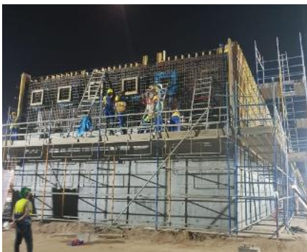
Left to right: thickener-tank reinforcement; slab pour at the chemical-dosing area; asphalt paving works.
