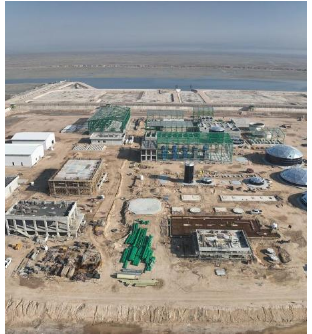
Main Outfall Drain (MOD) Water Treatment Plant, Basra — process tanks and treatment buildings under construction.
